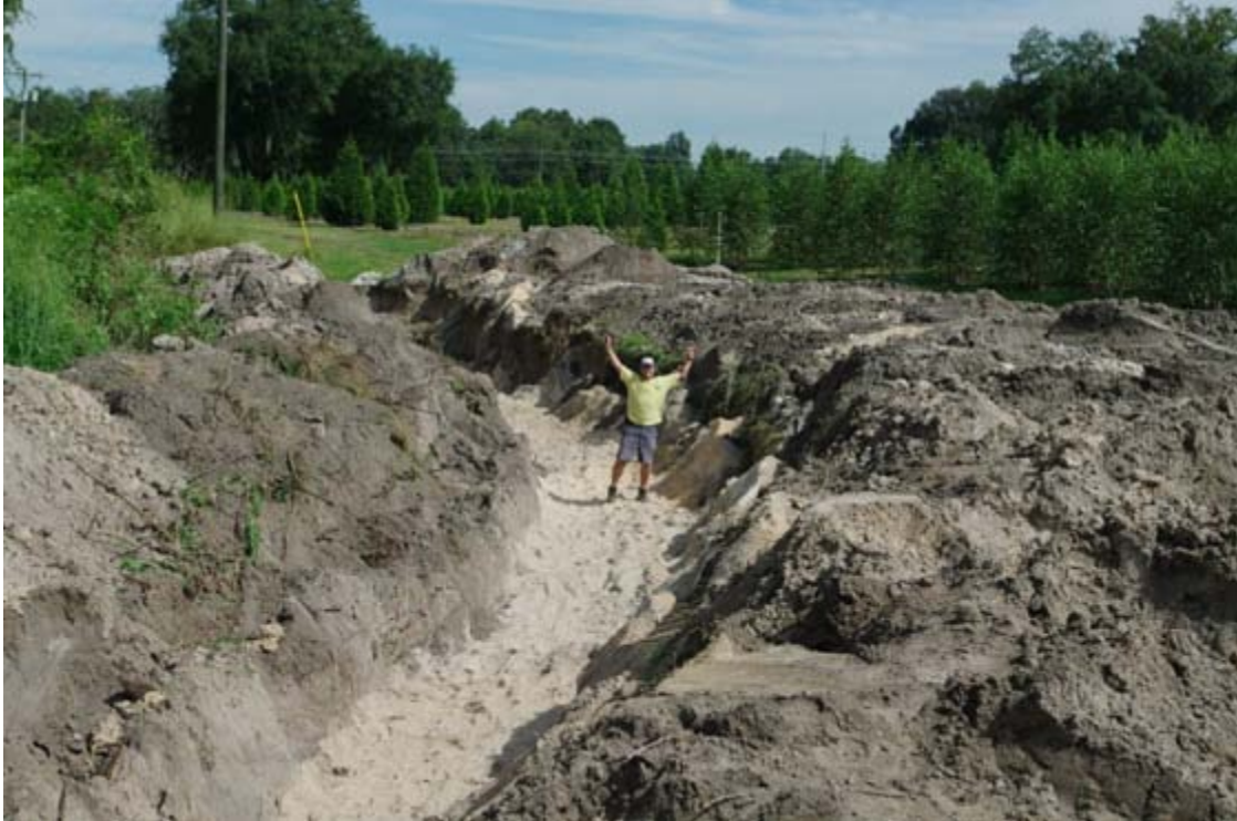
Figure 4-3. Excavation of denitrification wall trench (left) and backfilling with 50:50 sand:sawdust media (right)
