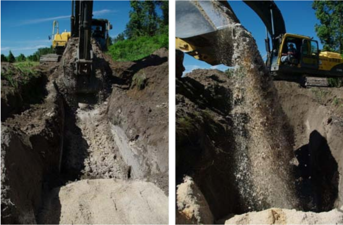
Figure 4-3. Excavation of denitrification wall trench (left) and backfilling with 50:50 sand:sawdust media (right)
