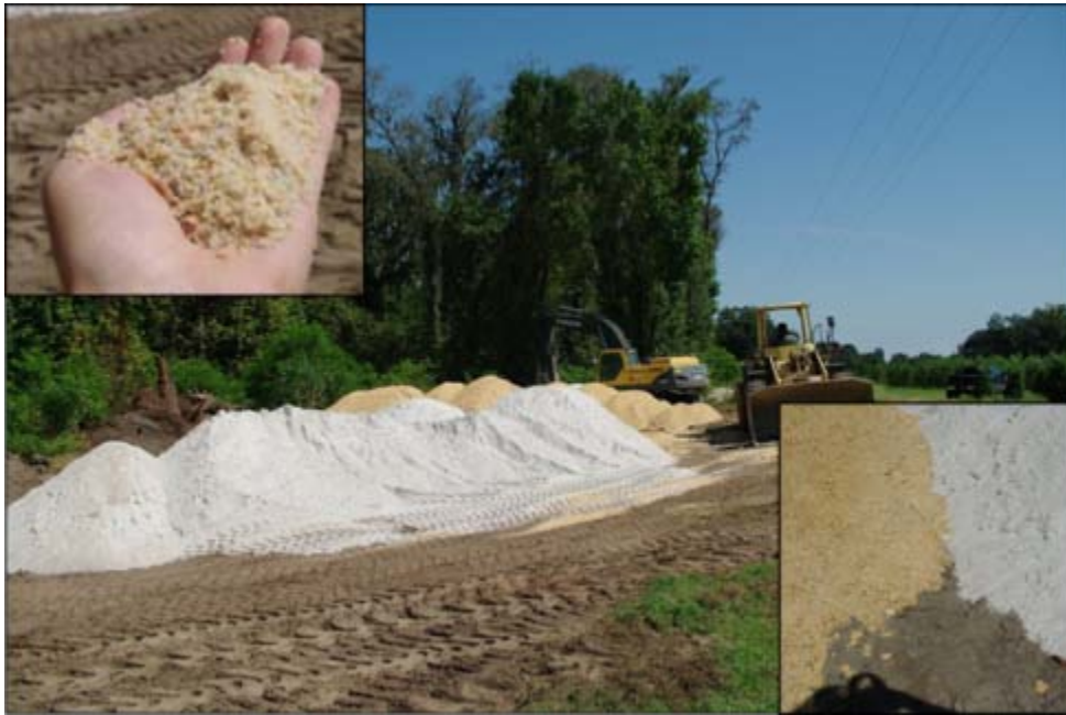
Figure 4-2. Sawdust and sieved quartz sand stockpiled in preparation for mixing and additional to denitrification wall trench. Image in upper left is photo of 50:50 sand sawdust after mixing.
