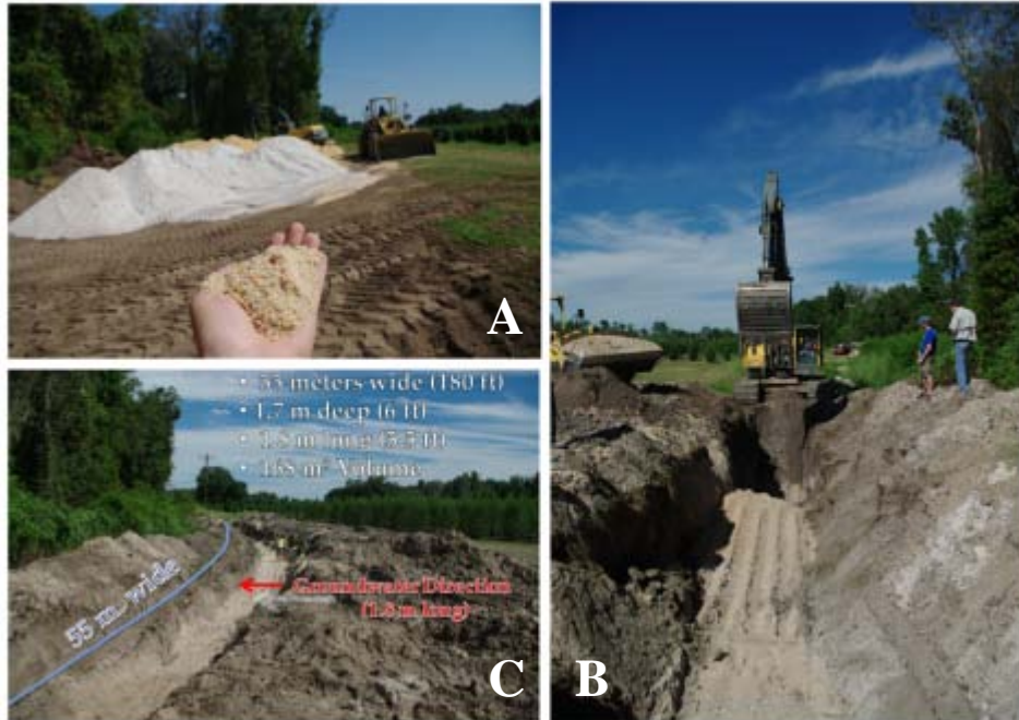
Figure 2 – (A) An image of the sand and sawdust used in the wall. (B) A trench was excavated to the desired depth and was immediately backfilled with the sand and sawdust mixture. (C) the final trench before backfill of surface soils.
