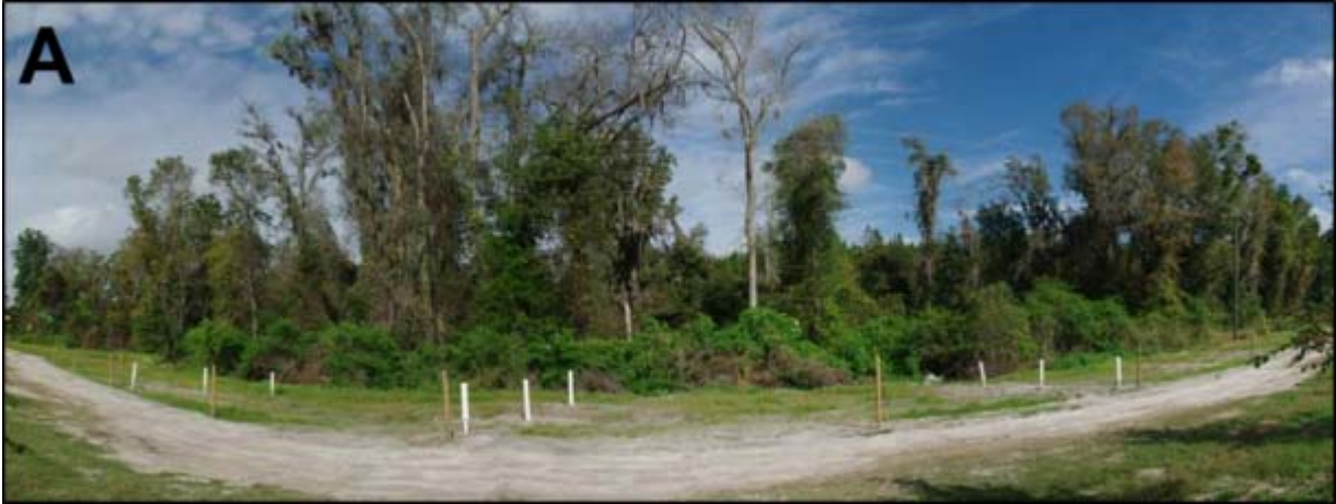
Figure 4-5. Completed denitrification wall with groundwater well transects the only evidence remaining of subsurface wall below. Flow is from foreground to tree line in background.
