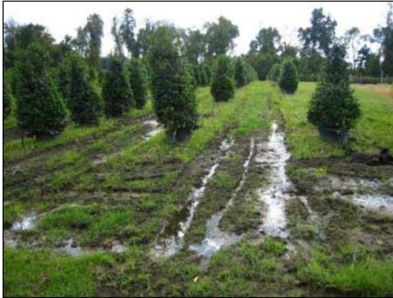
Figure 4-8. Area where well-drained surficial sands that occur in much of the rest of the nursery were absent and lower permeability clay soils are near the surface. The area already had poor production due to almost continuously saturated soils. The area was converted into a tailwater detention and treatment area as part of the BMP implementation effort.
