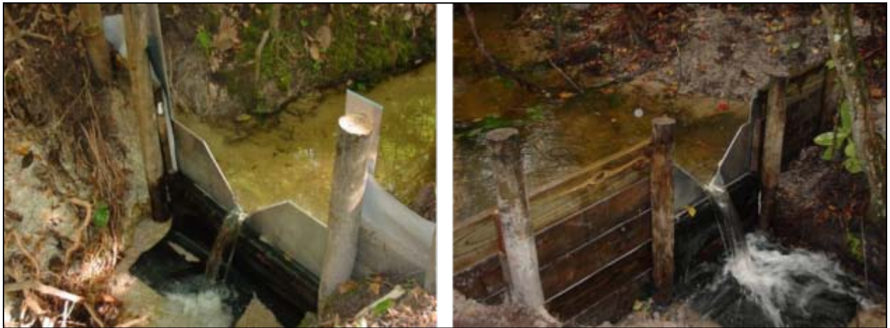
Figure 5-4 Compound weirs used to monitor the treatment watershed (left) and the control watershed (right)
