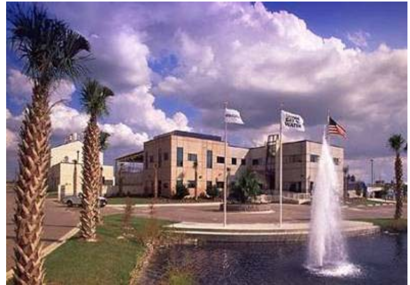
Regional Surface Water Treatment Plant
