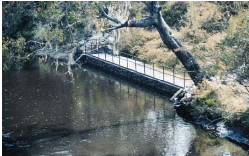
Alafia River Intake
