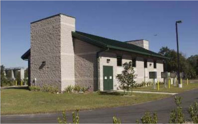
Tampa Bypass Canal
